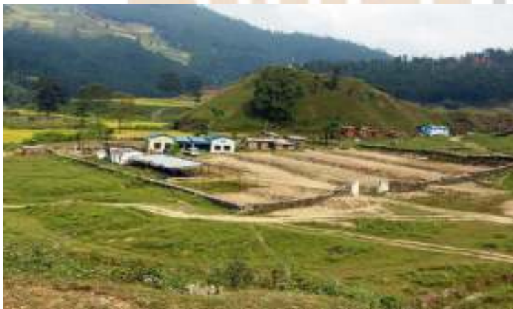
Fig 2: Oil drilling site of Dailekh
